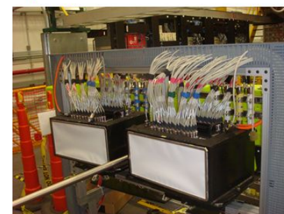
Status of Pair Spectrometer Installation
